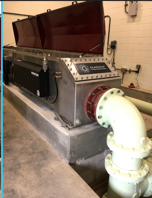
NONCON-5000 Installation. 3 MGD Plant. Remote Ballast Control Center with AB PLC Touch Screen OUI and Lamp Status Displays. glascouv.com NONCON-314-2018
