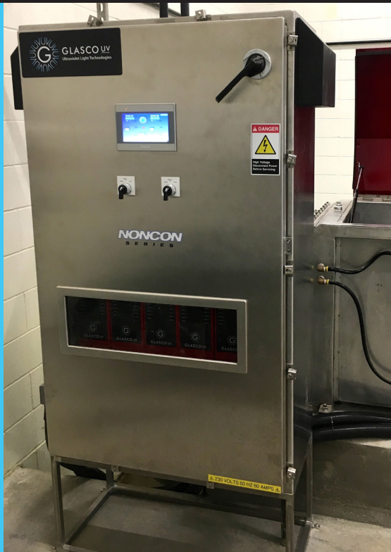
NONCON-5000 Installation. 3 MGD Plant. Remote Ballast Control Center with AB PLC Touch Screen OUI and Lamp Status Displays. glascouv.com NONCON-314-2018
