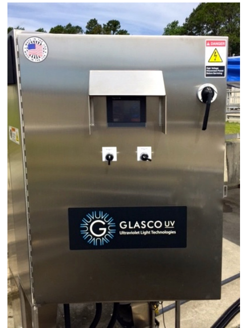
Replaced existing Power Distribution Center and provided flow pacing and added automatic quartz cleaning
