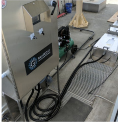
Replacement 2 x 2.5 MGD high output modules Installed Structure Above Channel
