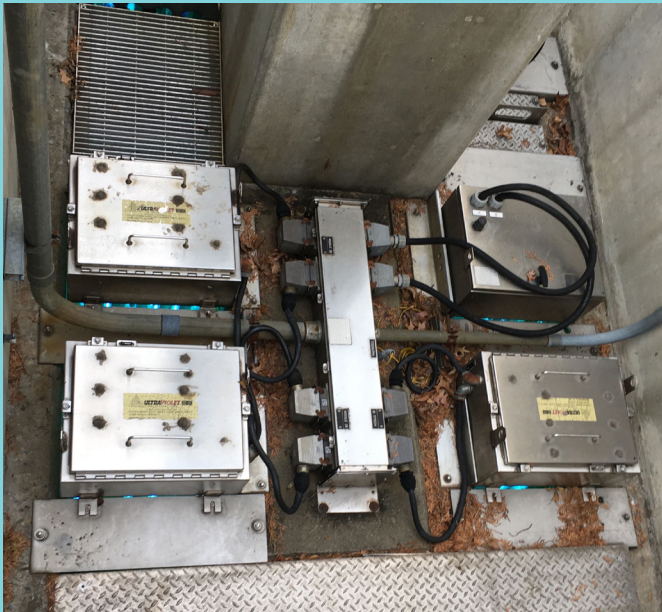
8 Module system using 320 low output lamps. No quartz cleaning or UV monitoring.
