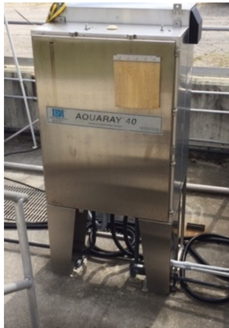
Replaced existing Power Distribution Center and provided flow pacing and added automatic quartz cleaning
