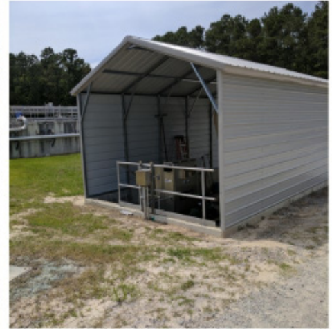
Replacement 2 x 2.5 MGD high output modules Installed Structure Above Channel
