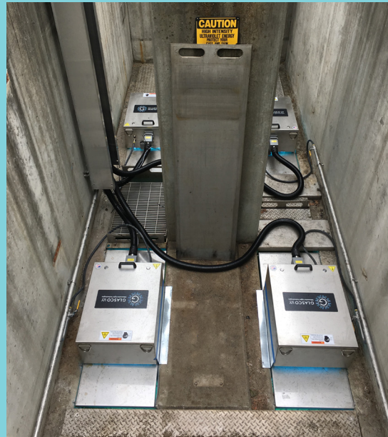
4 Module system using 96 amalgam UV-lamps. Added quartz sleeve cleaning and flow pacing. Matched footprint.
